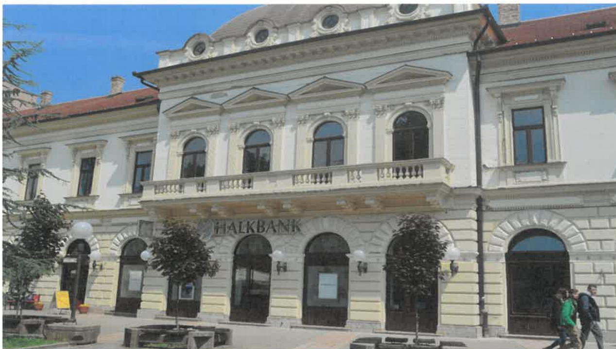
Halkbank's sub-branch in Pancevo
